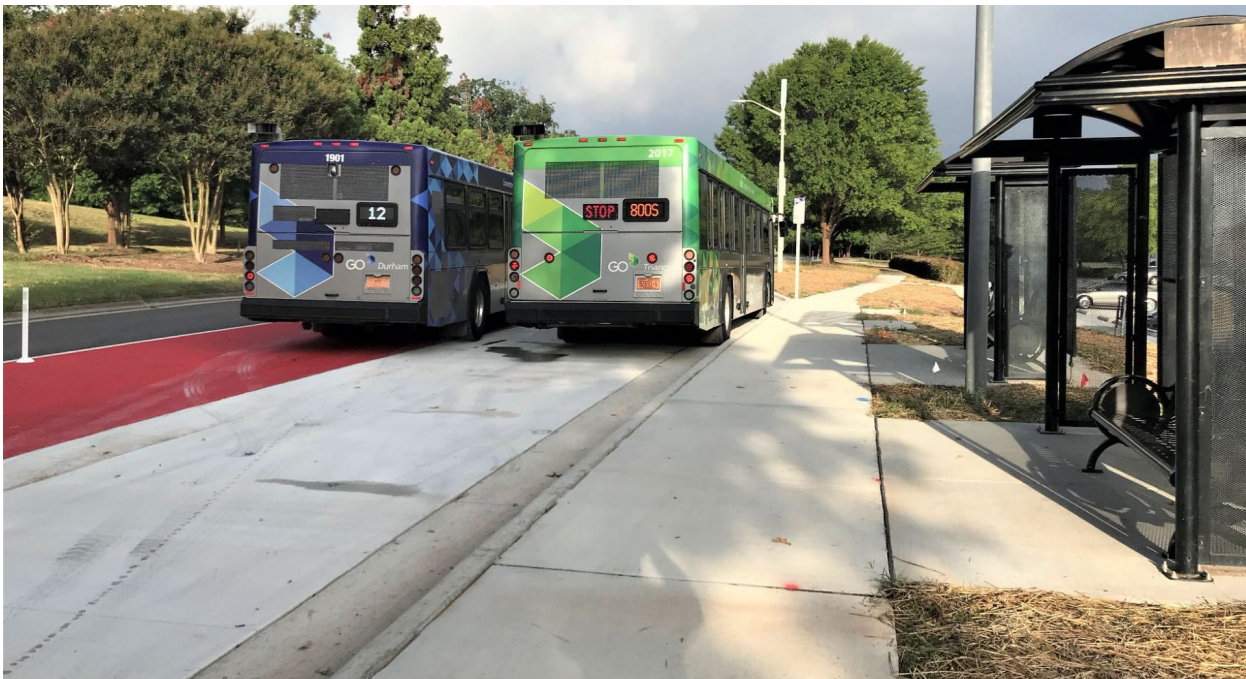
On Renaissance Parkway at Southpoint Mall in Durham, this stop was upfitted with two new shelters, benches, an ADA concrete pad, a bus bay, and a bus lane. It is served by both GoTriangle and GoDurham. (Source: GoTriangle)
